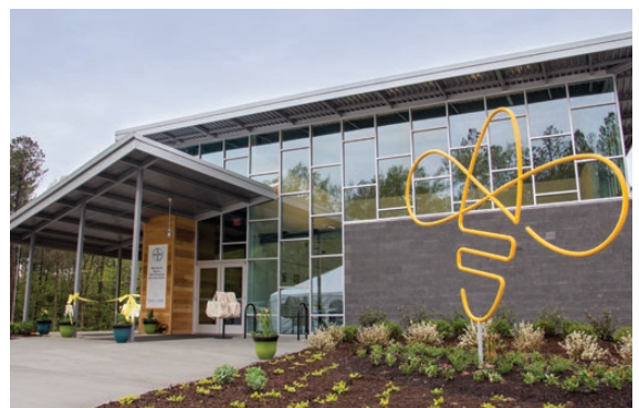
A 6,000-square-foot, state-of-the-art facility, Bayer CropScience's North American Bee Care Center comprises a honey extraction room, a hive workshop and an interactive educational room.
